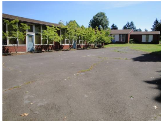
Southwest wing south elevation
