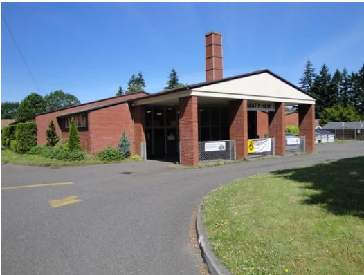
East elevation (cafeteria) front entry
